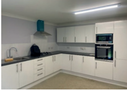
New Kitchen at Gliddon Drive. This is one of 9 new kitchens we installed in 2021/22
